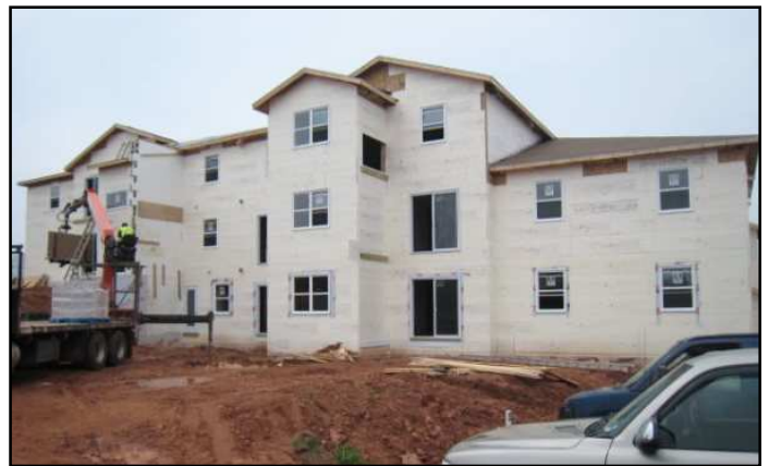
ICF Construction (concrete wrap under siding)
