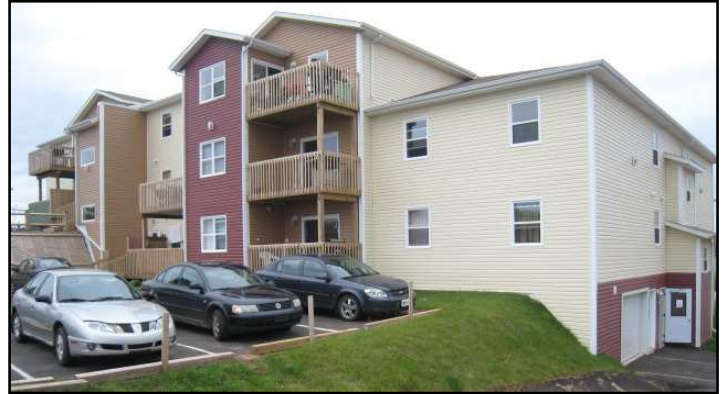
ICF Construction (concrete wrap under siding)
